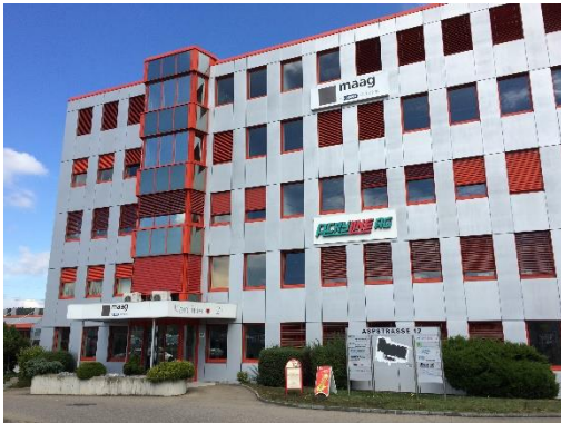
Photo: Maag corporate headquarters in Oberglatt, Switzerland
